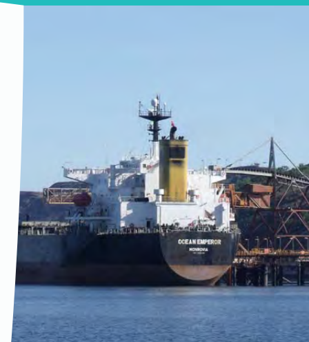
Loading at Koolan Island Photo: KLC
